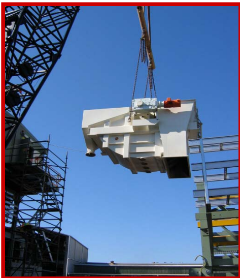
Filter without segments lifted into position in the filter building
