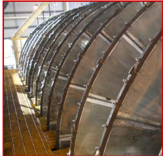
... and after revamping (improved access by permanent walkways)
